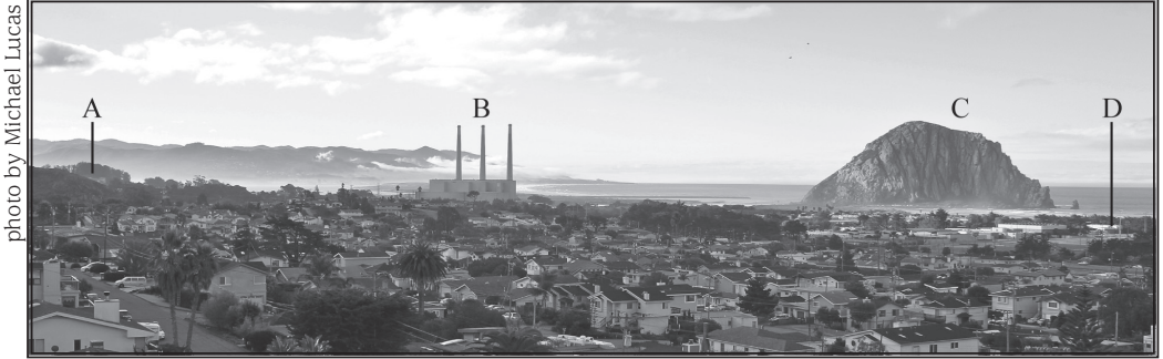
(A) Cerrito Peak; (B) Power Plant; (C) Morro Rock/Lesamo; (D) Water Waste Treatment Plant
